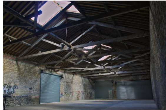
Internally showing shutters & skylights
